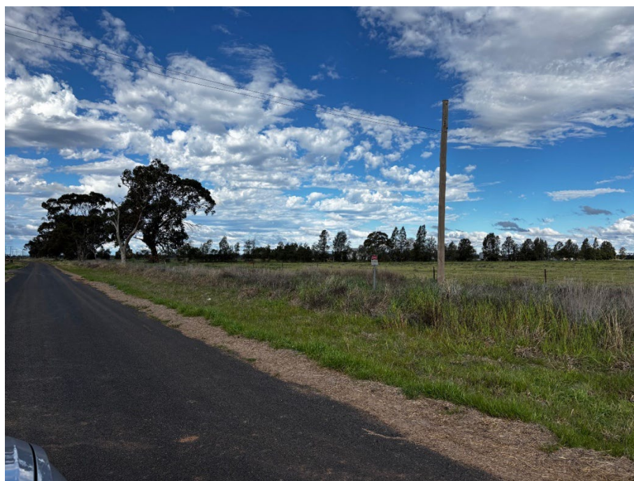
Figure 7: Gainsborough Road sealed western section with high pressure gas line on southern side of road reserve
