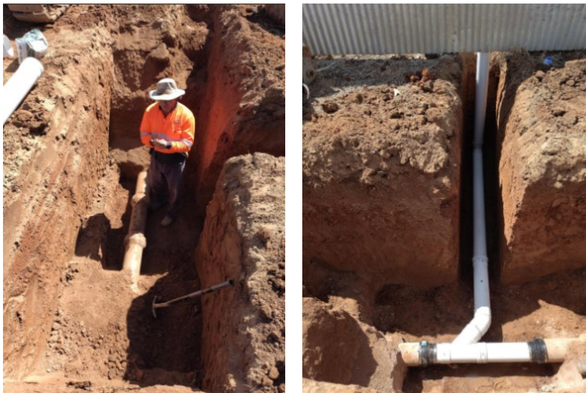
Figure 1: Installation of a sewer connection - Third Avenue
