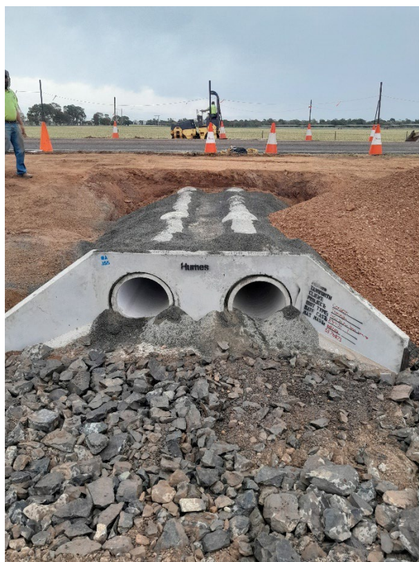
Figure 4: Culvert Extensions across Tomingley Road occurred in October
