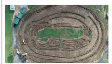
surface and sub surface drainage, installation of new irrigation and turf, new goal posts and boundary fencing to provide the community with a highly anticipated first class playing surface for the upcoming winter season.
